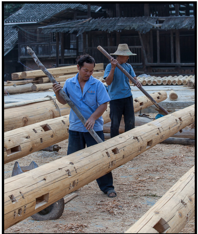
All joinery and construction is done this way, no nails and such.
