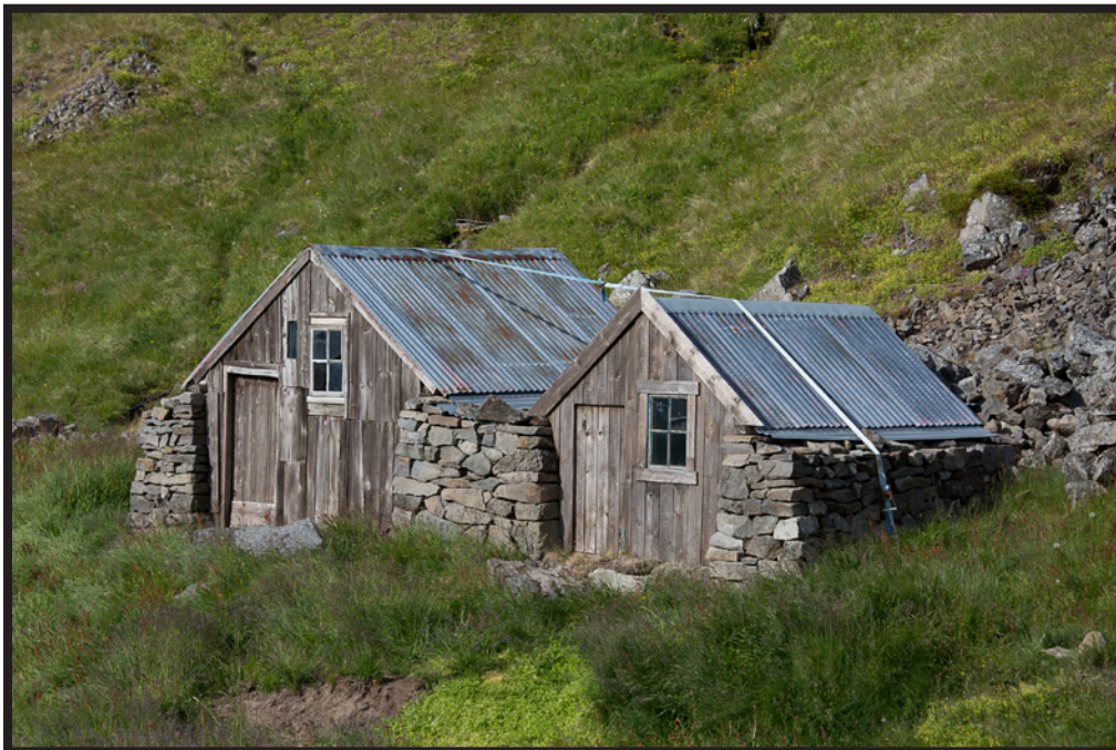
Roof hold down strapping indicates it may be windy at times?
